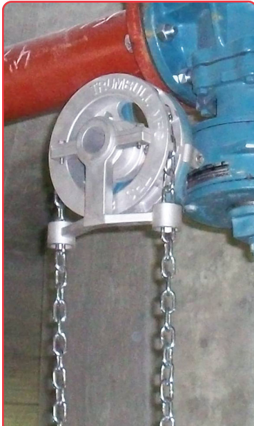
USED TO OPERATE OVERHEAD VALVES FROM THE FLOOR.
