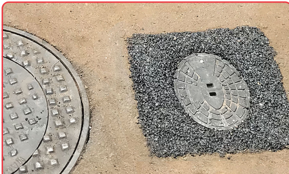
VAULT WITH REMOTE ANTENNA BOX.
