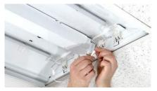
STEP 11: Adjust the LED boards to maximize your light beam spread.
