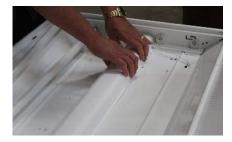
STEP 8: Connect the wire harness to the LED boards.
