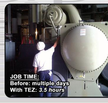
Above: This 2,000 ton chiller was pulled from atmosphe to 1,000 microns in only 3.5 hours, instead of days with belt-driven pump.
