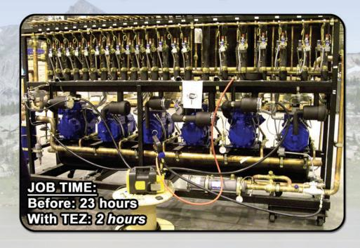
Above: With five simultaneous full-flow connections, the TEZ Speed System evacuates racks like these up to 10 times faster than typical vacuum pumps.
